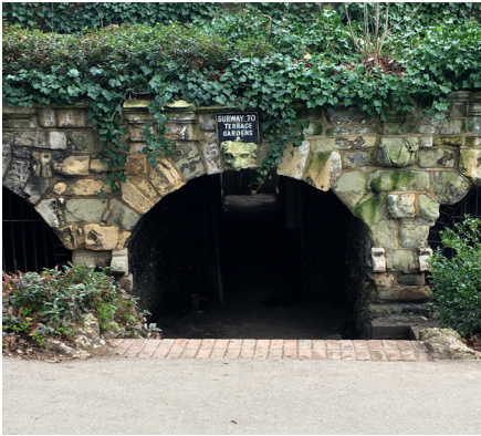
Subway under main road
