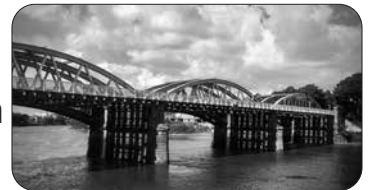
Barnes railway Bridge
